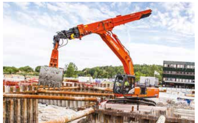
Special application excavators
